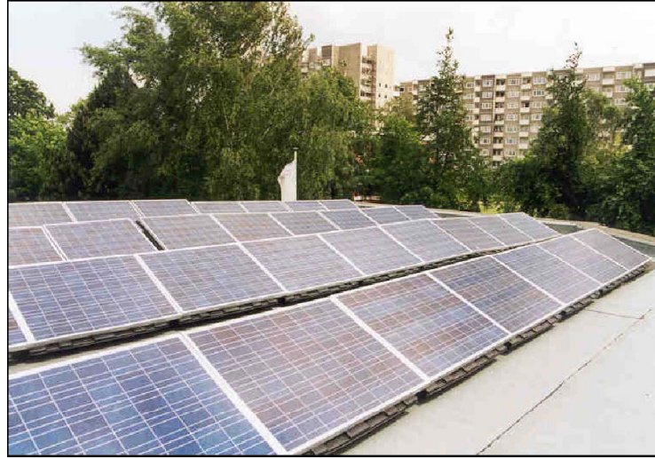
Photo 2.2: Example of installation on a flat roof (Goetzberger and Hoffmann, 2005)
